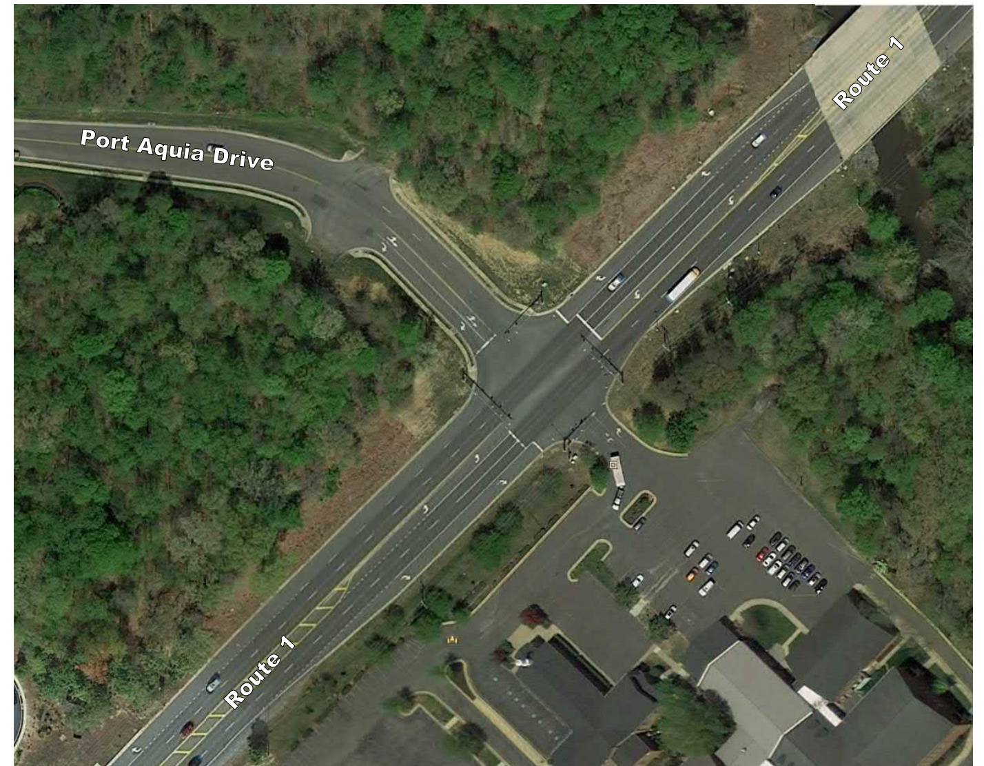
Figure 2: Route 1 at Port Aquia Drive
