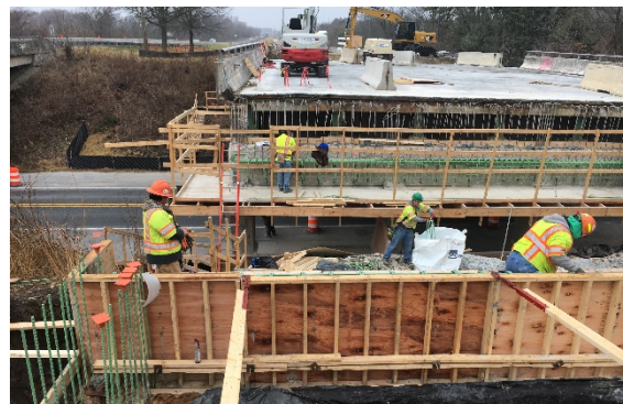
Installing rebar at Pier and formwork
