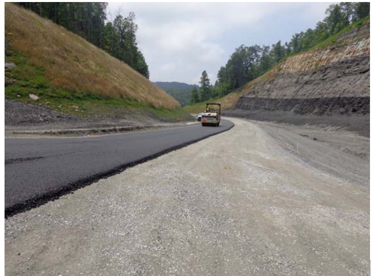
New US 460 Connector Roadway Pavement Placement
