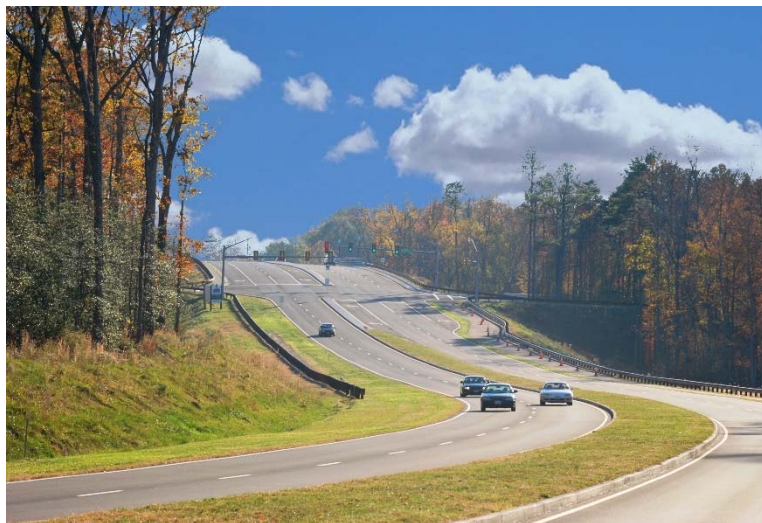
New alignment of North Gayton Rd. at the intersection of Bacova Dr.
