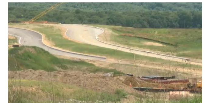
Relocated Southgate Drive (Route 314) under Construction
