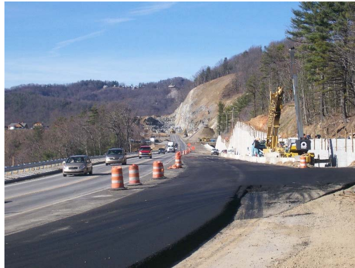
Paving and Retaining wall construction along Rte. 321
