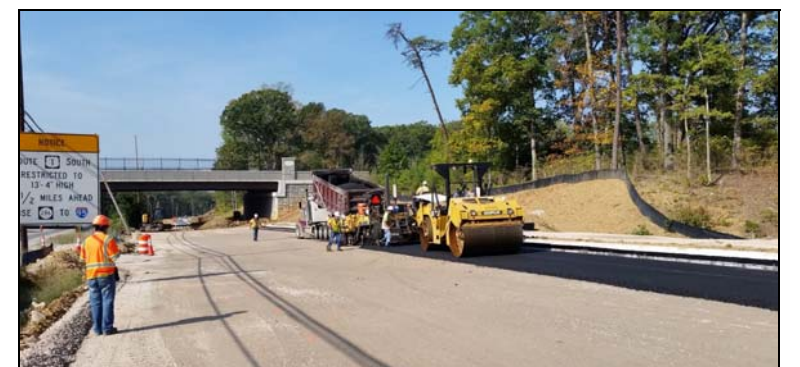
Route 1 Construction Progress Photos
