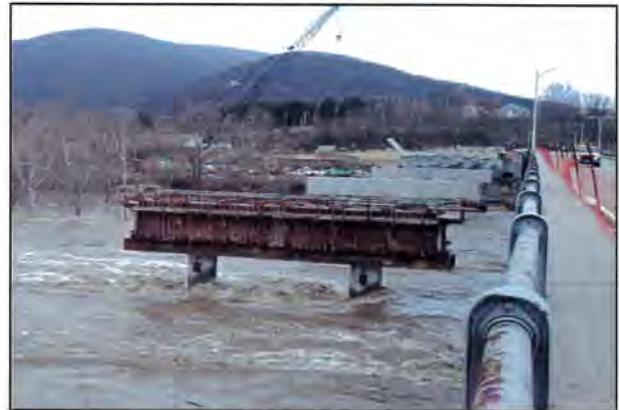
25-year Storm Event Presents Construction Challenge Route 61 over the New River
