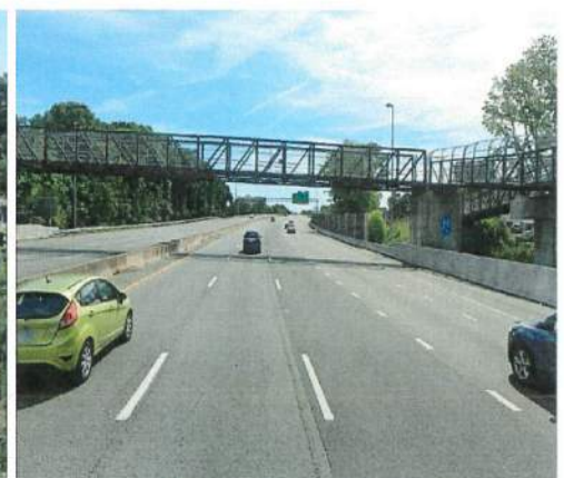
MLK Pedestrian Bridge City of Portsmouth, VA
